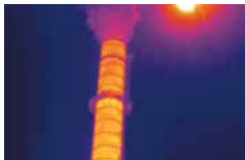
Refractory material inspection on a furnace chimney.
