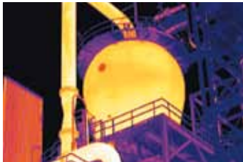
Refractory insulation inspection on a petrochemical reactor
