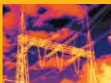
Inspection of high voltage power lines
