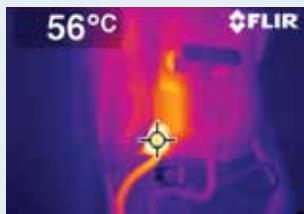
What a thermal imaging camera sees.
