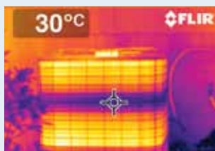
What a thermal imaging camera sees.
