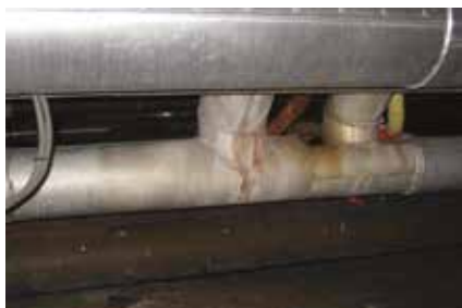
Visual and thermal image of one of the pipes in the network. The thermal image clearly shows imperfect insulation.
