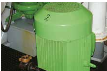
Visual and thermal image of an electric engine driving a pump in a tanker engine room.
