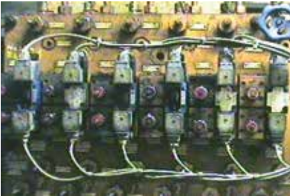
Visual and thermal image of a defective control module (second from right).
