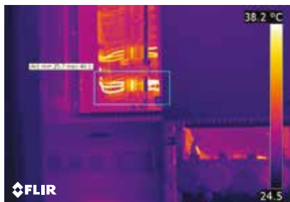
Although these output terminals are definitely hot, the measured temperatures are normal for this kind of load.
