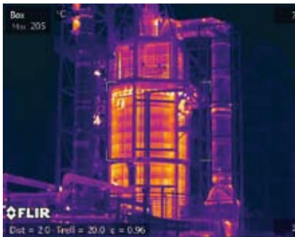
Infrared image of a process furnace
