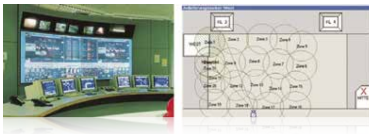
Figure 7. Control room for waste pile processing, and screen capture of the zone monitoring layout, which uses a FLIR IR camera on a pan-tilt mount for fire hazard warning.
