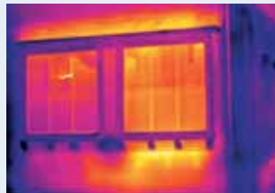
What a thermal imaging camera sees.
