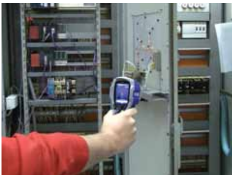
The students are trained to distinguish between real hot spots and reflections.
