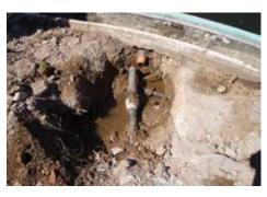
The repair workers were directed to open up the pavement where leaks were inspected, to find broken or cracked pipework, validating the results from the thermographic survey.
