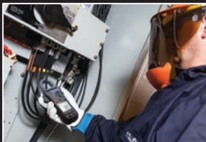
Analyze power-related issues
